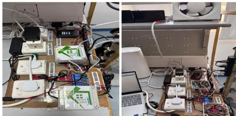
Fig. 5. Particle Photon-driven Environmental and Air Quality Control Subsystem (PPEAQCS) prototype
